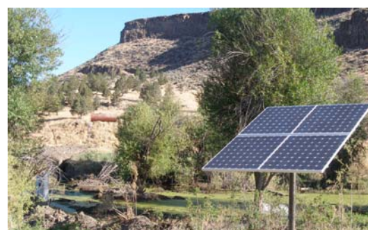
Figure 2. A 600 watt solar array running a 95 liter per minute pump to provide off stream water to 400 pair of beef cattle in a rotational grazing system.
