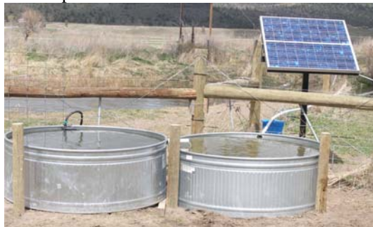
Figure 1. A 160 watt solar array powering a 13.3 liter per minute pump providing off stream water to 25 horses and 35 sheep.
